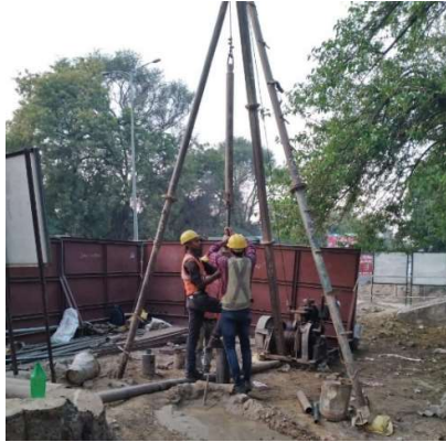
Fig. 3. Borehole in progress
