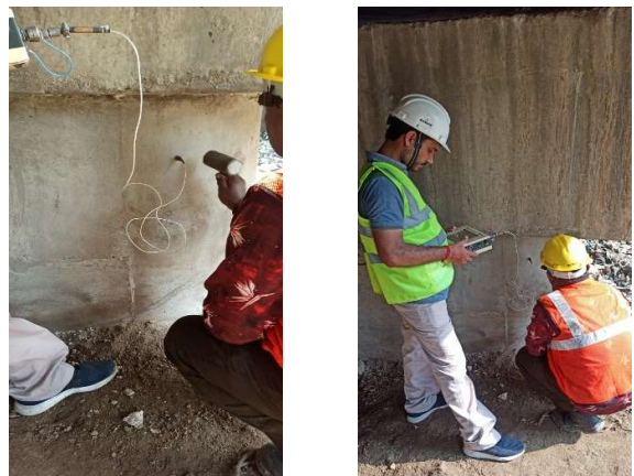
Fig. 5. Sonic pulse-echo test in progress on the underside of the bridge
